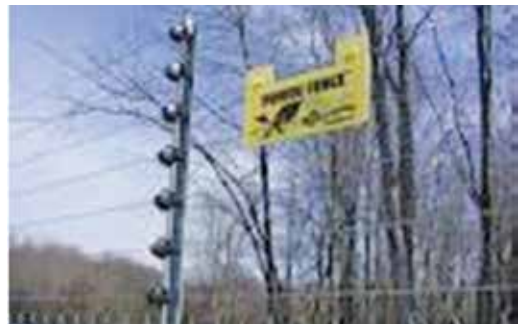
Fig. 6 Electrified Fence
