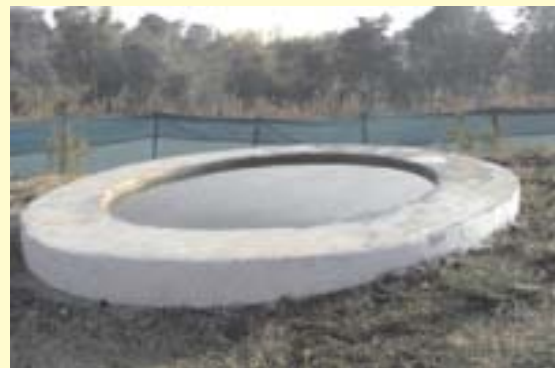
Water storage tank in nursery
