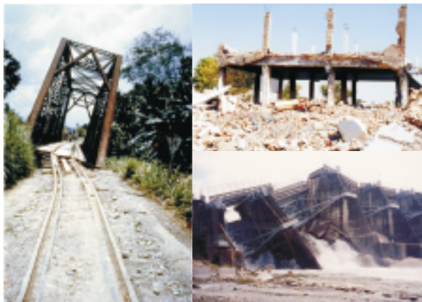
Fig 2.1.4 shows the adverse effects of an earthquake
