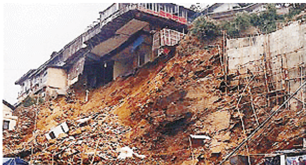
Fig 2.6.1 Landslide in hilly terrain of India
