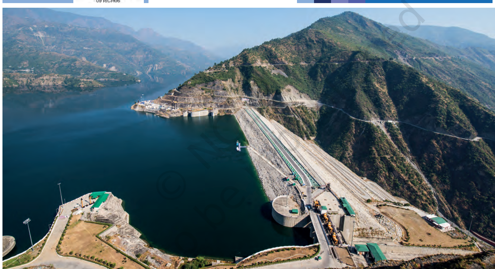
Figure 6.1: Tehri dam in Uttarakhand
