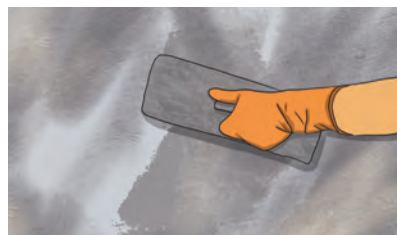
Figure 6.19: Applying plaster on the wall
