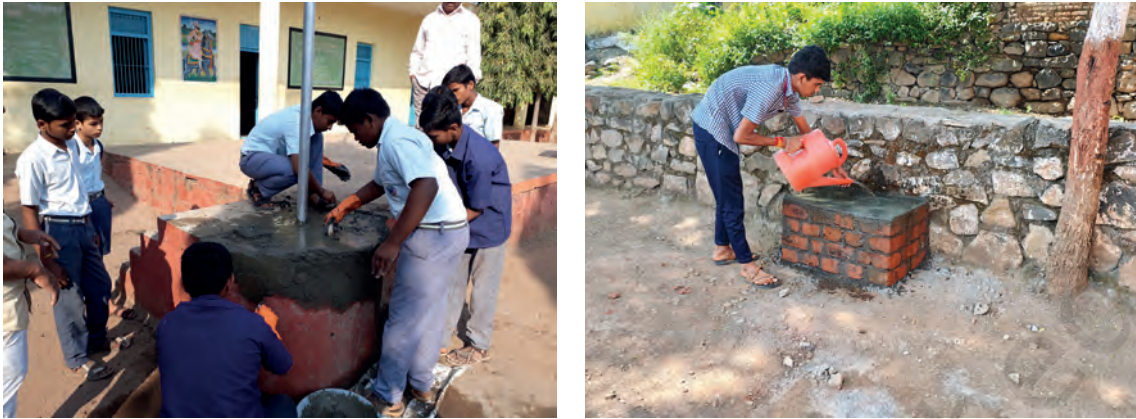
Figure 6.22: Structures built by students
