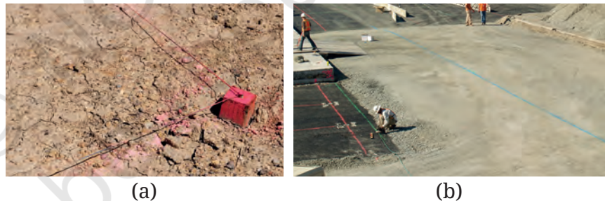
Figure 6.13: (a) Using reference lines for marking site of construction, and (b) marking lines for construction
