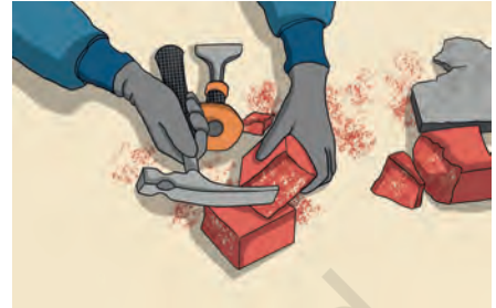
Figure 6.16: Cutting the brick using chisel and hammer
