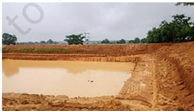
Figure 5.13: Percolation tank for groundwater recharge
