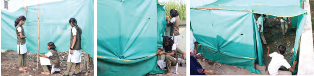
Figure 1.10: Installing the green shade-net
